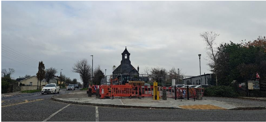
PEDESTRIAN CROSSING UPGRADE WORKS HAVE COMMENCED AT CREAGH CHURCH JUNCTION, BALLINASLOE
