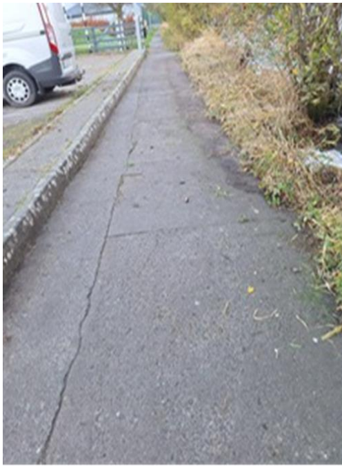
..... CLEANING FOORPATH AT LOUGHREA LAKE AND PLAYGROUND
