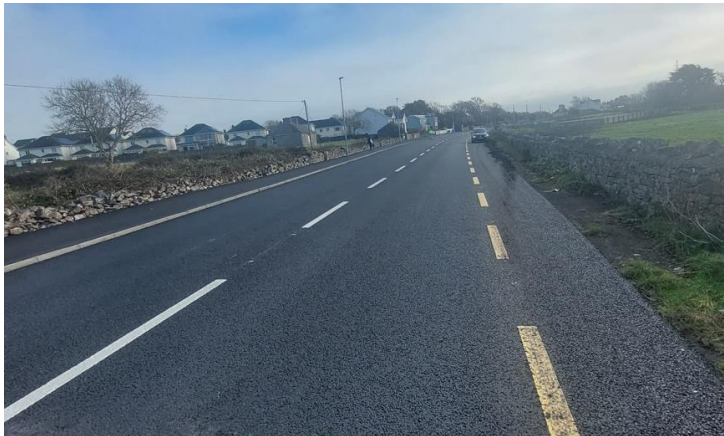
COAST ROAD FOOTPATH AND ROADWORKS
