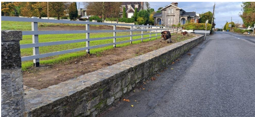
COMPLETED CIS PROJECT AT DÚN ÍDA, BALLINASLOE
