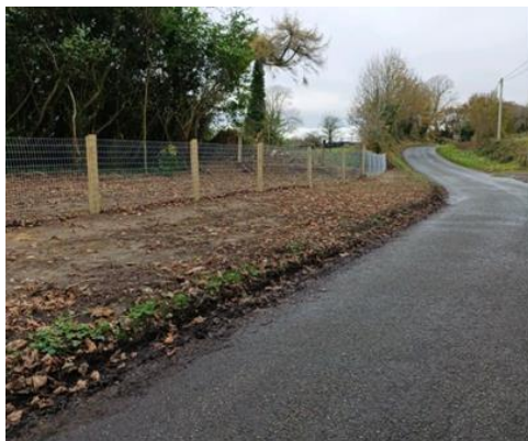
DRAINAGE WORKS BELWELL
