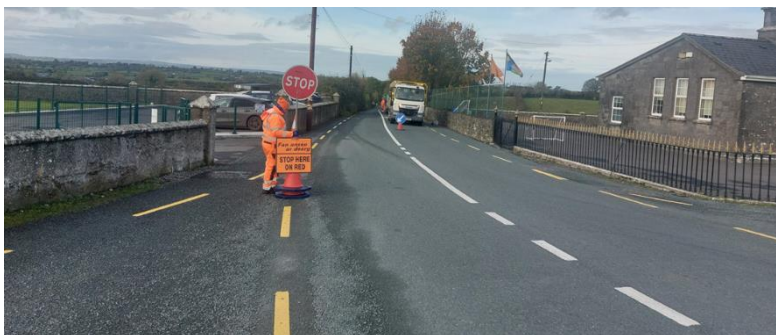
ROAD RELINING AT GORTANUMMERA NATIONAL SCHOOL
