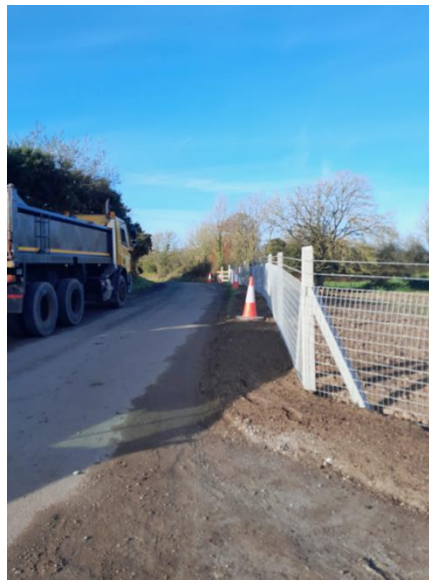
PRE AND POST WORKS AT LISHEENY, ABBEY TO IMPROVE SIGHTLINES AT BEND
