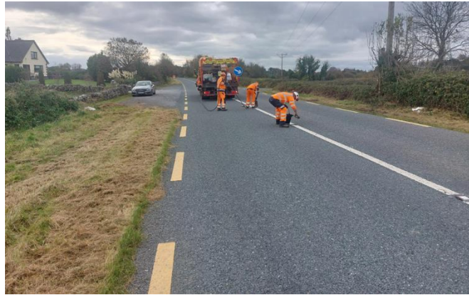
INSERTION OF NEW REFLECTIVE STUDS "CATS-EYES" ON THE R458
