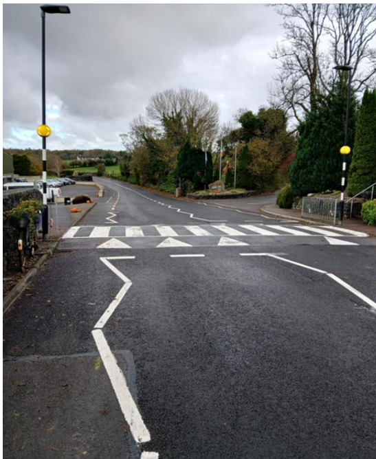
AN FHAIRCHE - RESTORATION IMPROVEMENT WORKS
