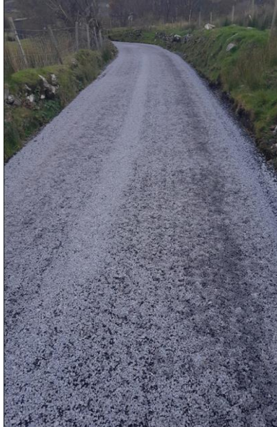
RECENT LOCAL IMPROVEMENT WORKS - BEFORE AND AFTER
